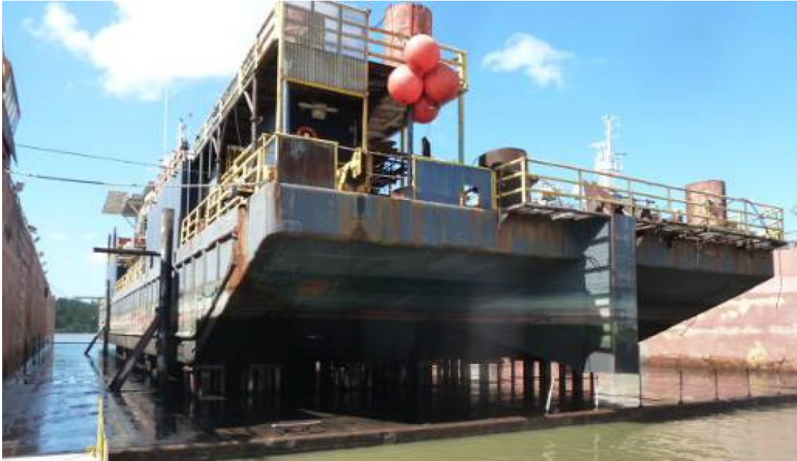
Rider Pipelay barge
